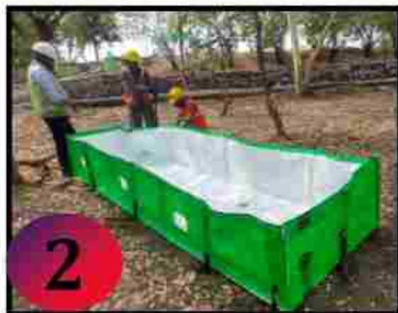
2 Erection of Vermi Bed
