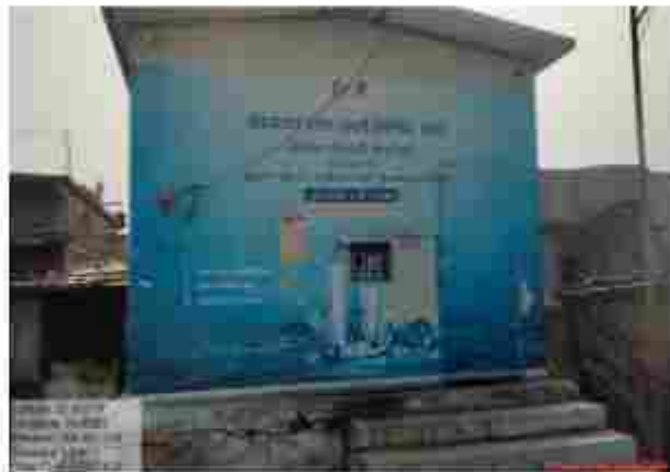
R.O. WATER PLANT
